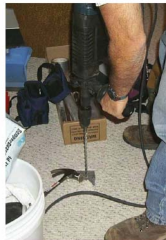
Figure 1. Drilling through a slab
